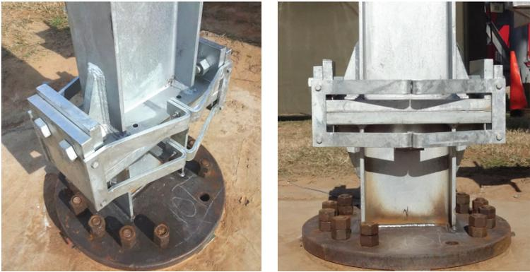
Figure 1.5 High capacity moment collar breakaway connection developed in FDOT project BDV31-977-24
